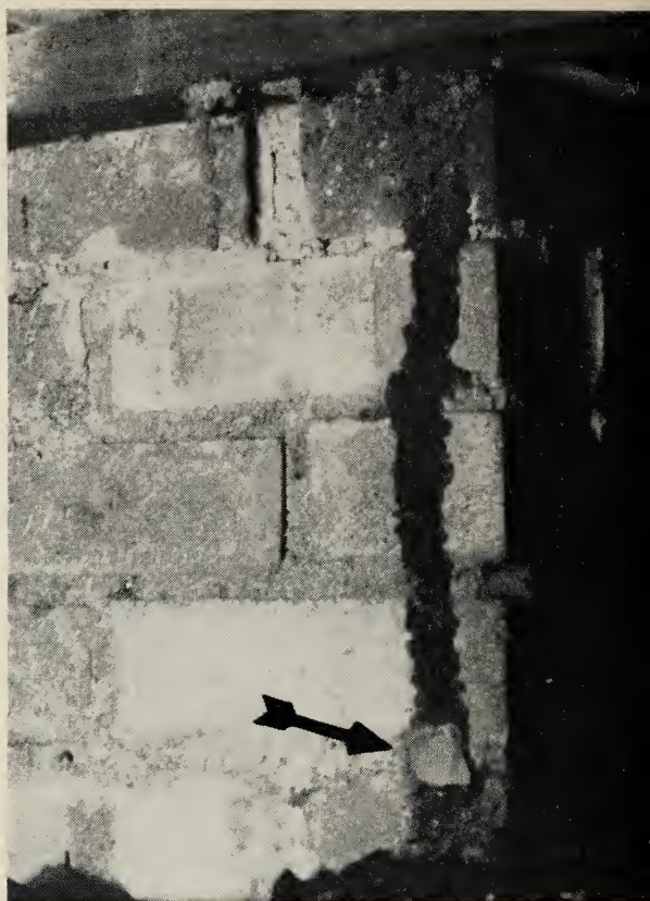
Fig. 14. Main shelter tube of Coptotermes acinaciformis connecting ground and floor joist. Note paper pasted over hole into which arsenic dust was blown. (From Casimir, 1957.)
